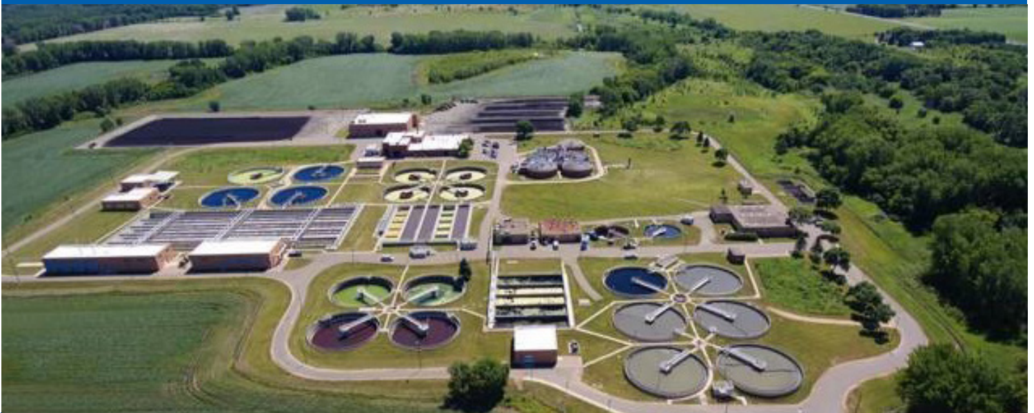
MCES Empire Wastewater Treatment Plant
