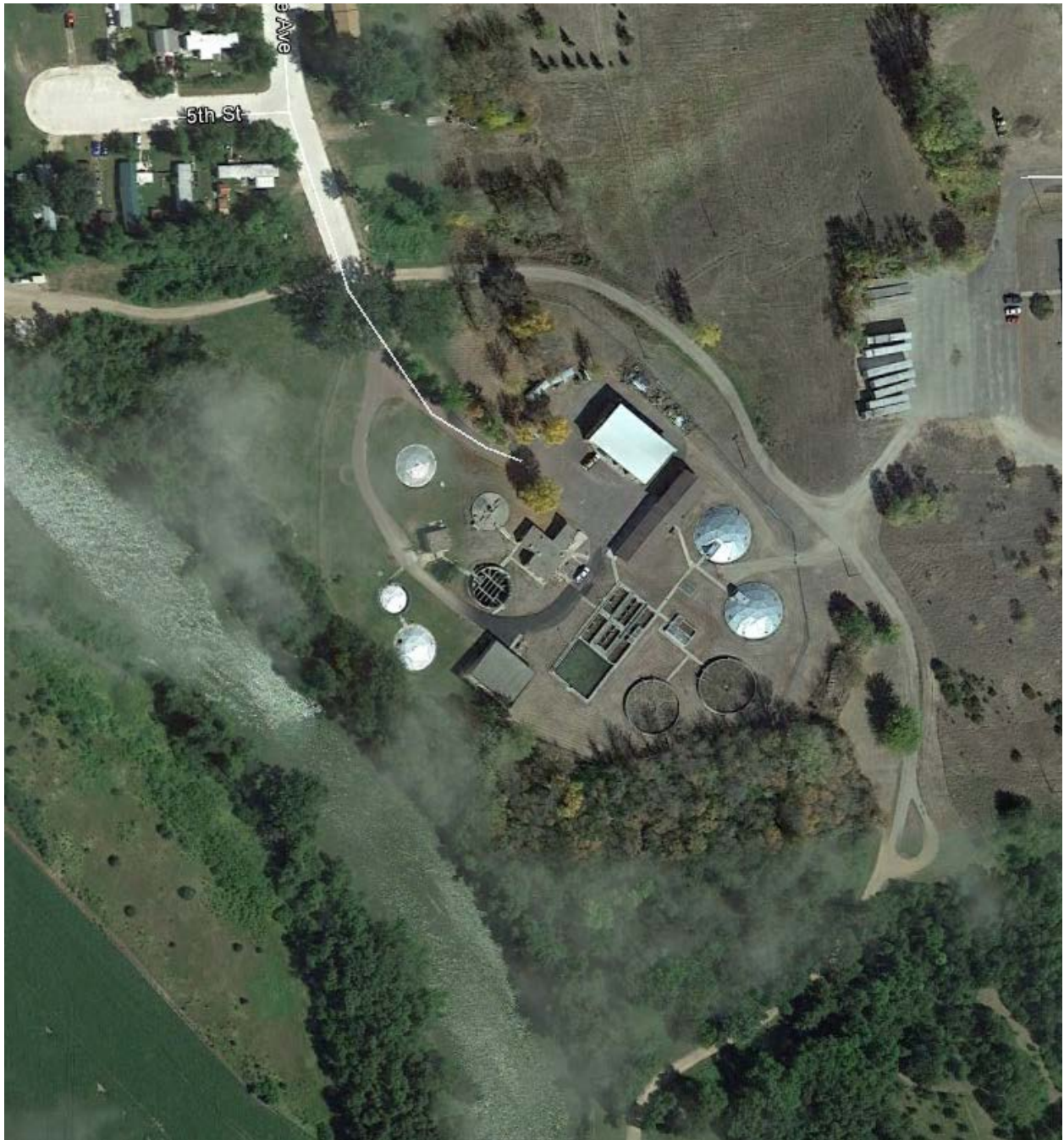
Figure 3.1. Windom WWTF Aerial Overview
