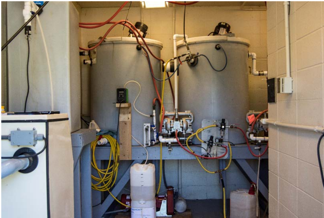
Figure 4.4 Pilot Scale 2-Stage Activated Sludge Construction (pre-anoxic and aeration basins).
