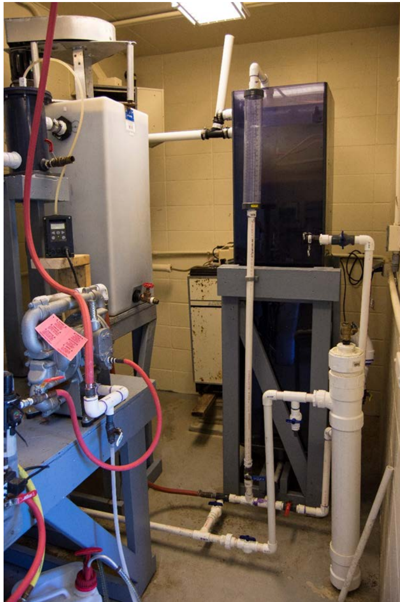
Figure 4.5 Pilot Scale 2-Stage Activated Sludge Construction (post-anoxic and clarifier).
