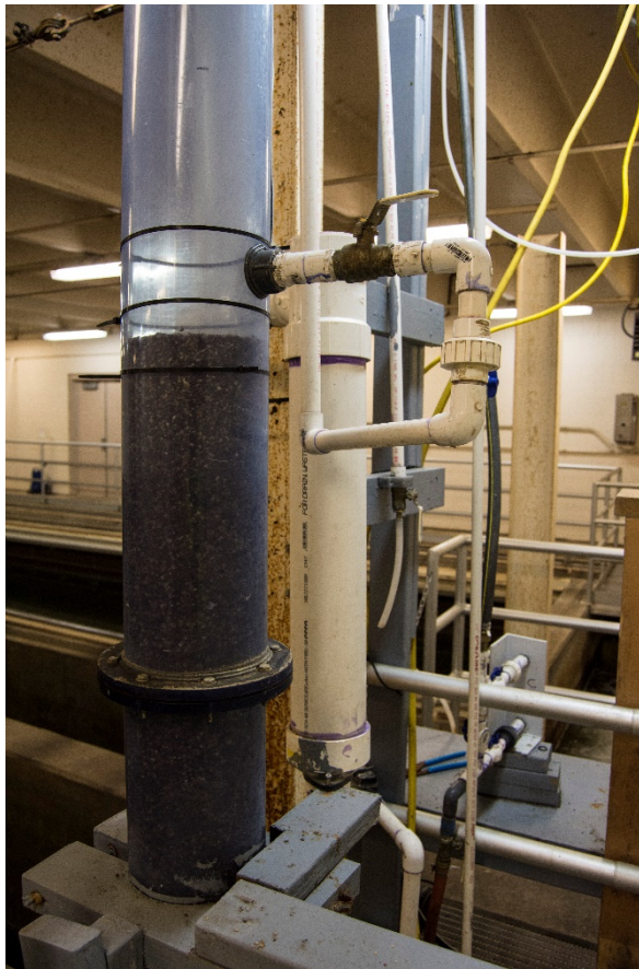
Figure 4.2 Pilot Scale Denitrification Filter System Construction
