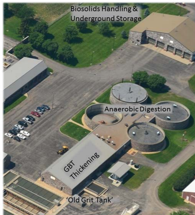
Figure 3. Solids handling at St. Cloud WWTF
