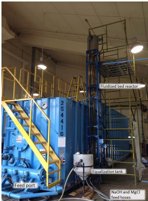
Figure 7. Ostara reactor set up at St. Cloud WWTF in Biosolids handling building.
