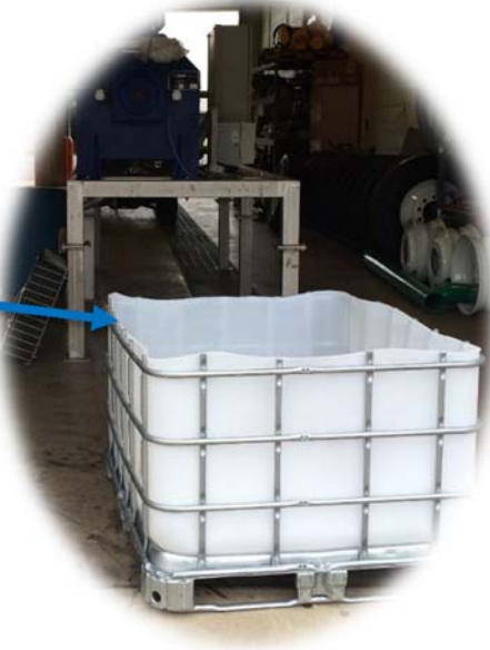
Figure 18. Recycled tote cut in half was used as a wet well and a sump pump and flat hose were used to transfer from end of screw-press to holding tanks.
