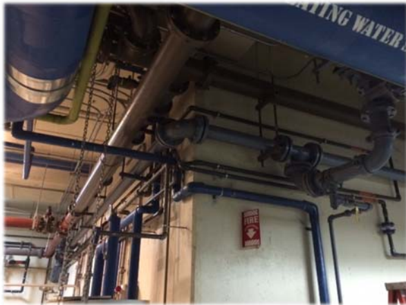
Figure 12. Reconfiguration on basement piping enabled enclosed transfer of waste activated sludge (WAS) from final clarification tanks to the un-used grit tanks to fermentation.
