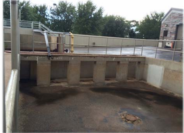
Figure 12. Reconfiguration on basement piping enabled enclosed transfer of waste activated sludge (WAS) from final clarification tanks to the un-used grit tanks to fermentation.
