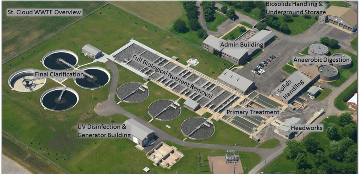
Figure 2. St. Cloud WWTF Overview.
