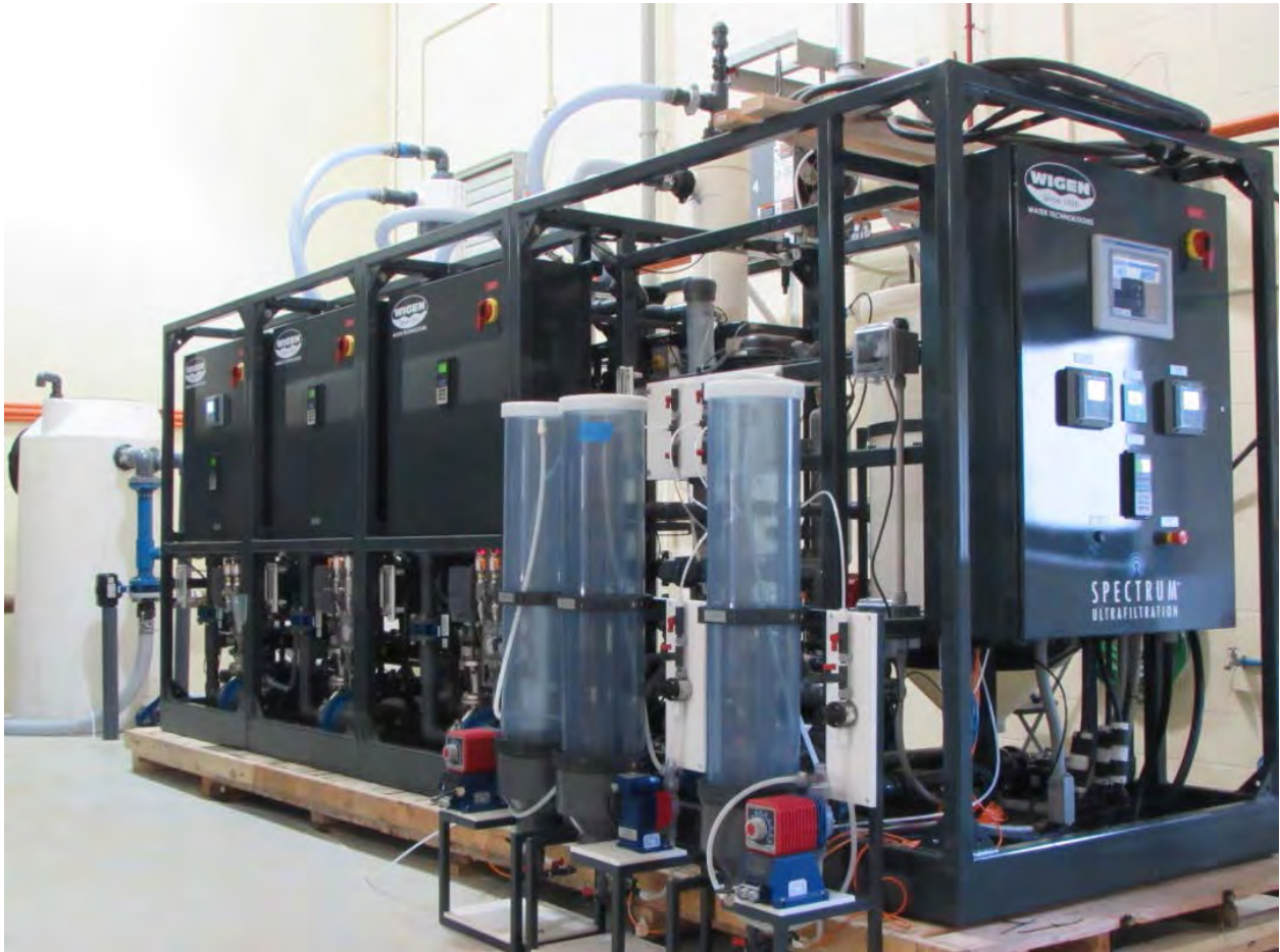
Figure 3.4.1: UF Pilot Skid utilized at the Mankato, MN Pilot study
