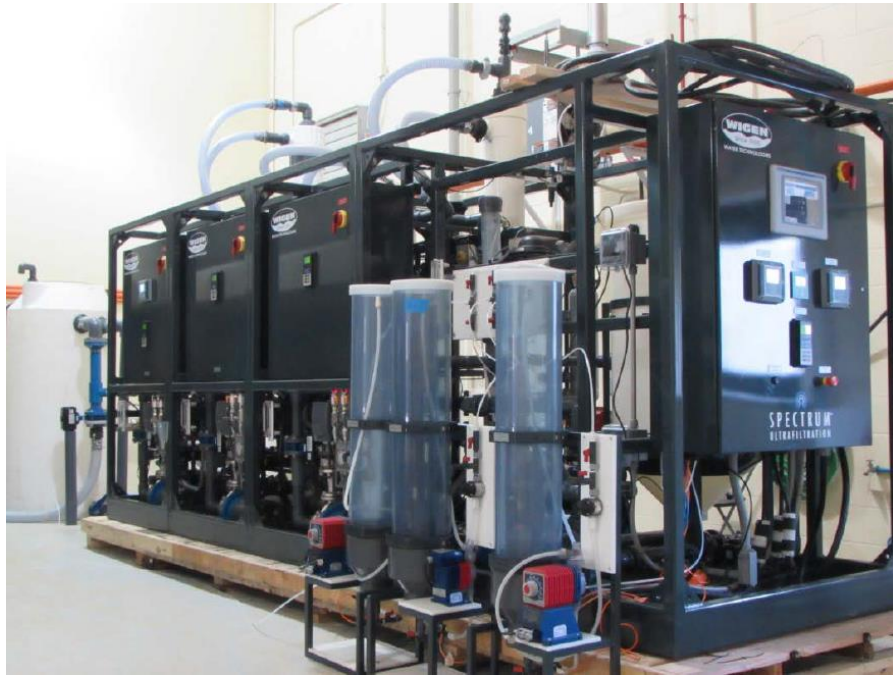
Figure 4.2 – Photo of Ultrafiltration Pilot Skid (Wigen)
