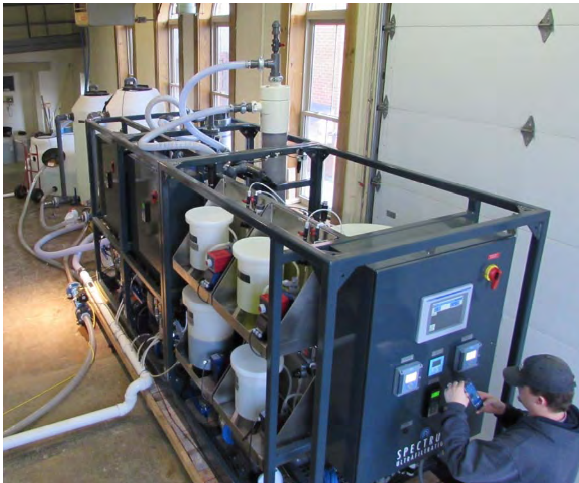
Figure 1: UF Pilot Skid Proposed for Study (Feed and backwash tanks at rear).
