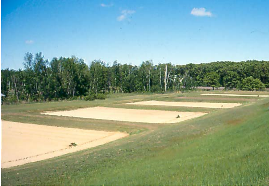
Figure 1: Rapid Infiltration Basins.
