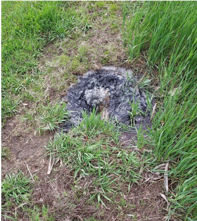
Figure 22. Sewage discharging to the surface.
