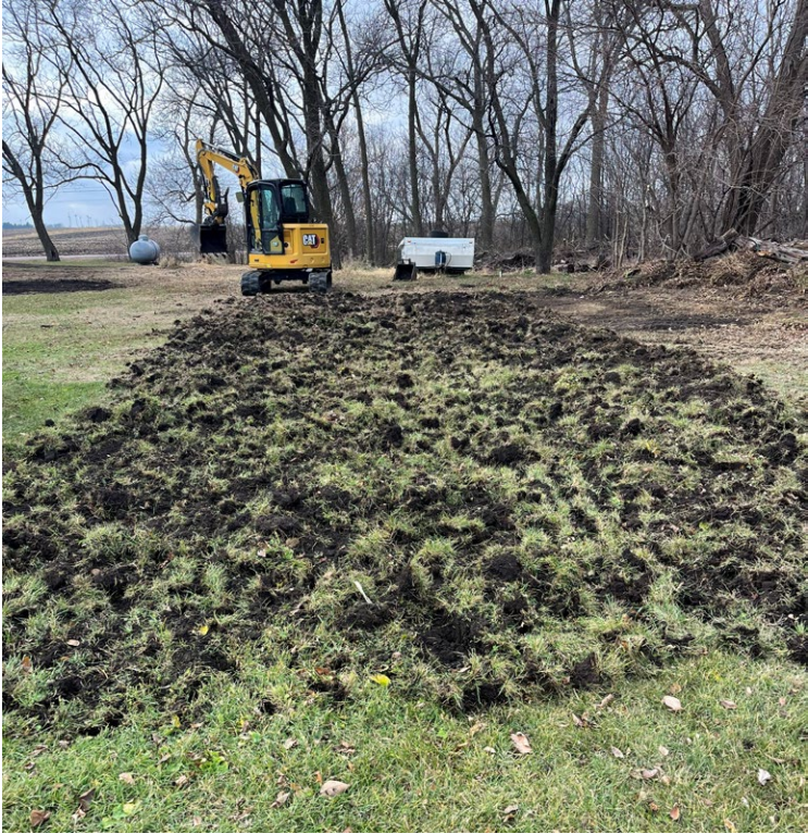
Figure 4. Photo of the original soil mound absorption area roughened.
