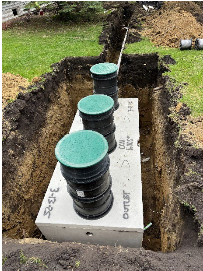
Figure 12. New concrete tanks being installed.
