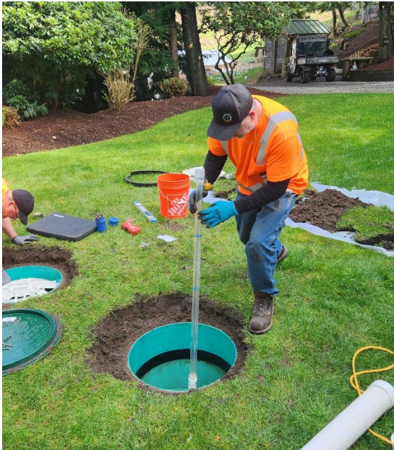
Figure 8. Measuring sludge and scum in septic tank.
