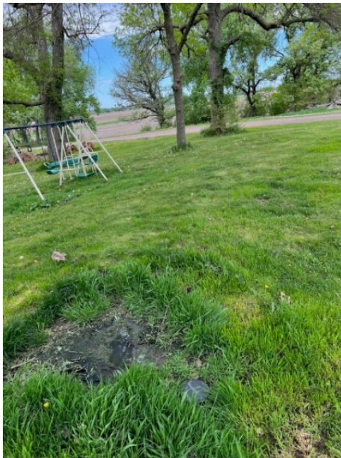
Figure 22. Sewage discharging to the surface.
