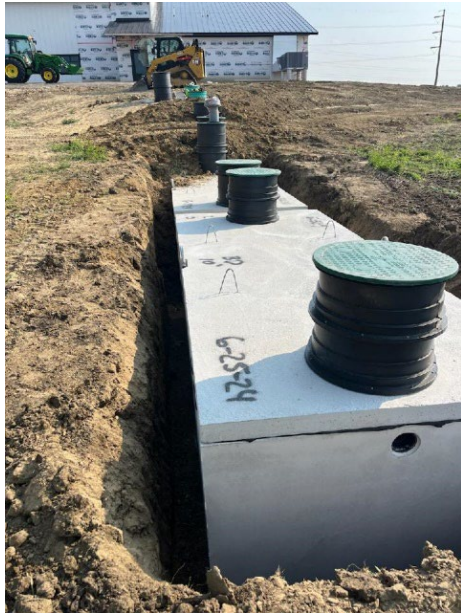
Figure 12. New concrete tanks being installed
