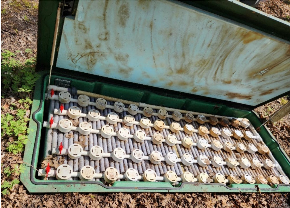
Figure 7. Type IV system using a registered proprietary treatment product of a fixed media filter.
