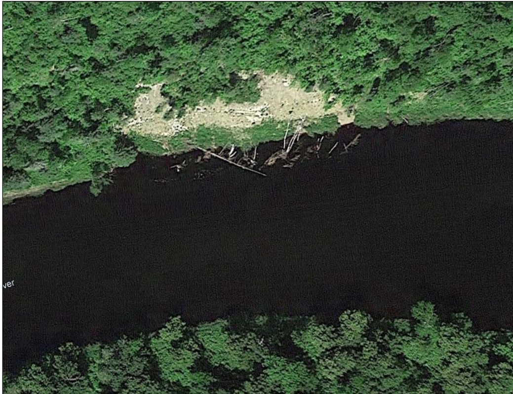
Figure 23. Another example of bank failure on the Big Fork River. The trees that toppled from the bank can be seen below the failure in the water.
