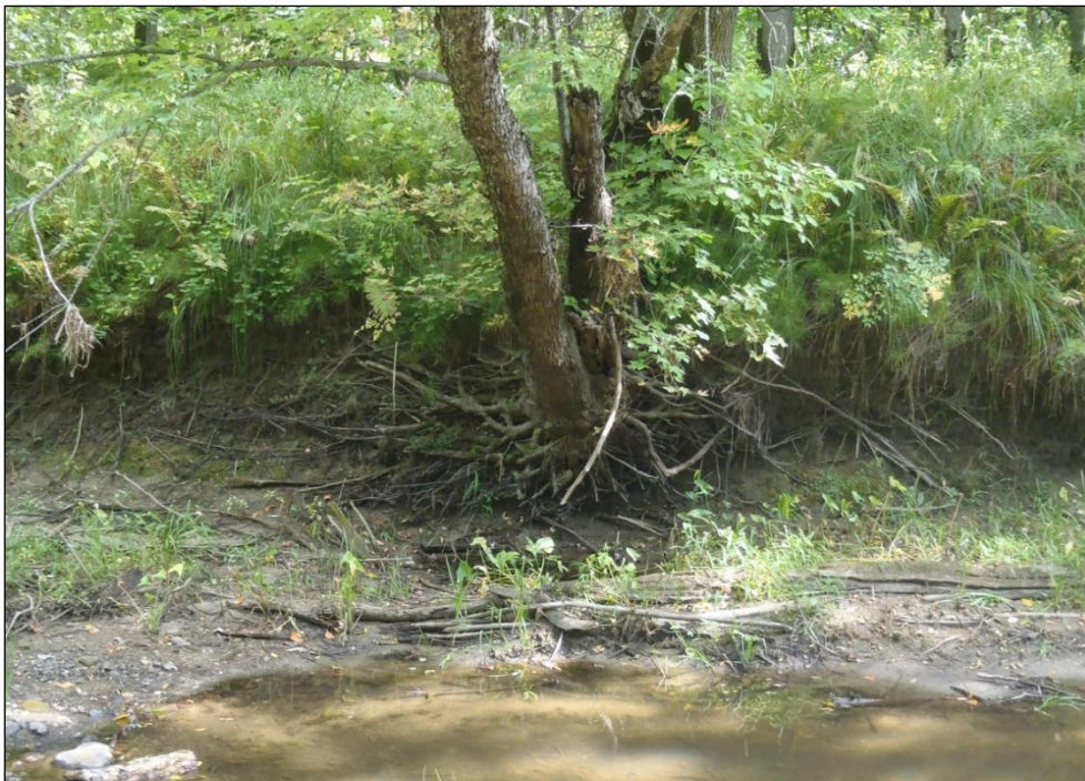
Figure 16. A bank tree that has been completely undermined by erosion and is now down in the stream channel with most of its roots exposed, soon to be a contributor to one of the many log jams seen on aerial photos.
