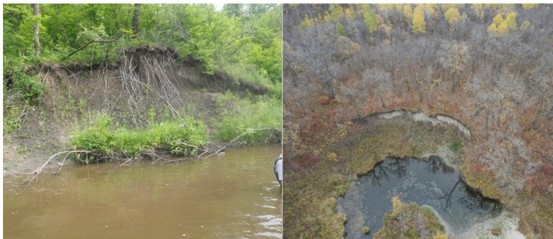
Figure 4. Images of bank erosion along the Black River (AUID 09020303-529), including Station 12RD002 on June 13, 2012 (left), and near Site S002-132 (CSAH 18 crossing) on October 14, 2025 (right).
