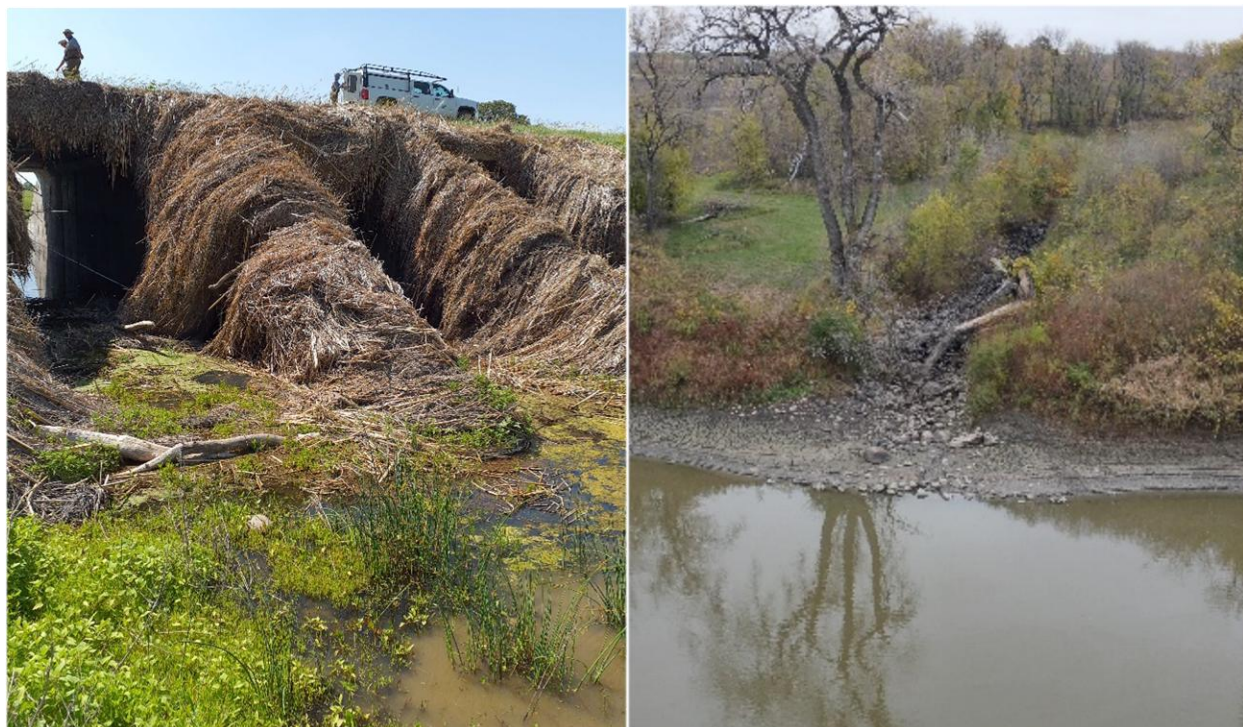
Figure 16. Flow-related images for Grand Marais Creek (AUID 09020306-530), including low flow conditions and vegetative debris deposited during a prior high flow event at Station 23RD009 (CSAH 64 crossing) on June 20, 2023 (left), and a dry streambed at the outlet to the Red River of the North on October 15, 2025 (right).
