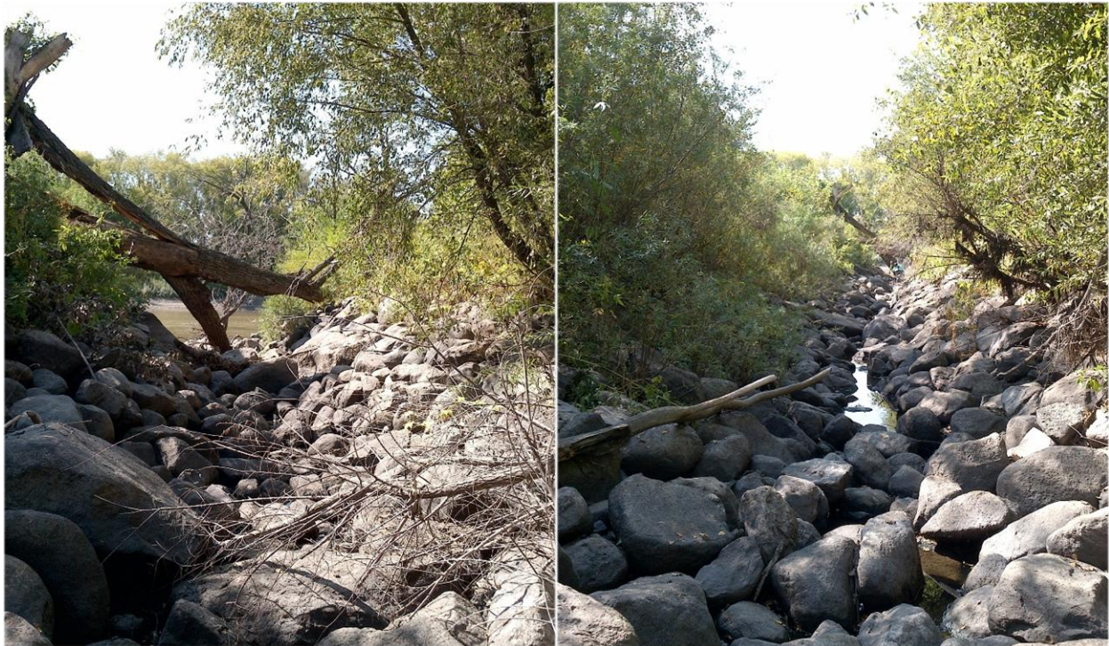
Figure 13. Images of riprap within the channel of Grand Marais Creek (AUID 09020306-530) near its outlet to the Red River of the North on September 16, 2025; images courtesy of the DNR.
