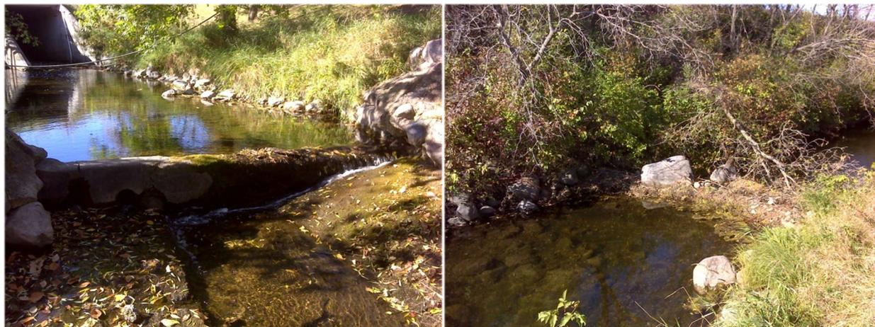
Figure 51. Photos of potential connectivity barriers along AUID 554 on October 8, 2014, including a small concrete dam immediately downstream of the CR 11 crossing (left) and a beaver dam downstream of the 180<sup>th</sup> Avenue SW crossing (right).
