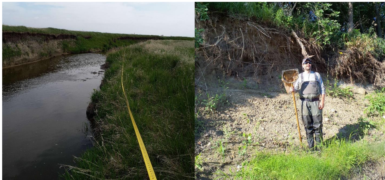
Figure 3. Images of bank erosion along the Mustinka River, including Station 10RD034 (near State Hwy 9; AUID 09020102-582) on May 19, 2021 (left) and Station 21RD075 (near CSAH 11; AUID 09020102-583) on August 4, 2022 (right).
