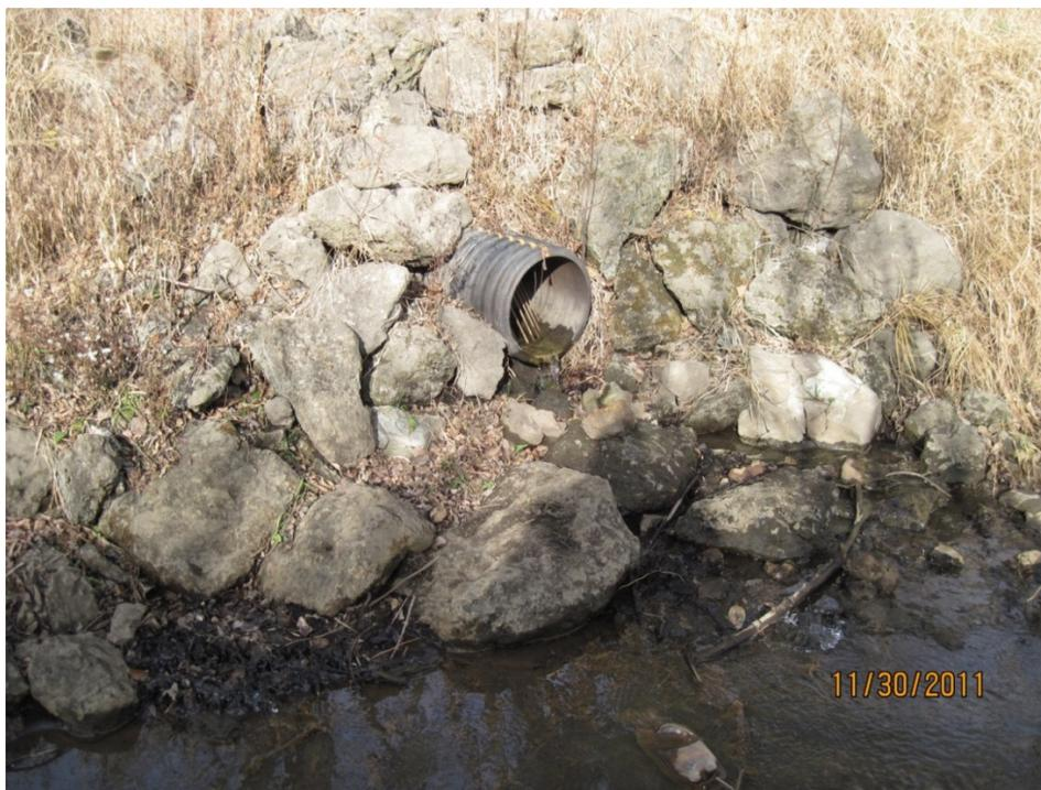
Figure 10: Example of a drain tile outlet to a stream in the Cedar River Watershed.
