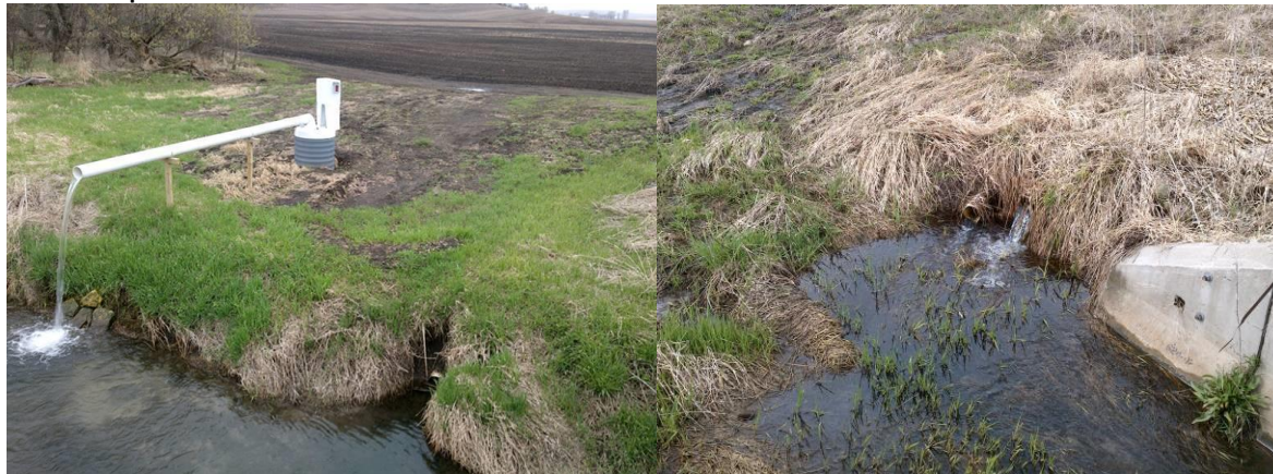
Figure 18. Various photos of tile drainage in the area of nitrate increase. Left photo: lift station and streamside tile both contribute to tile water at various times of the year. On 7/22/22, the streamside tile was sampled with a result of 19.5 mg/L. Right photo: Multiple tiles contribute to a tributary that had an average concentration of 12 mg/L, as determined from 9 samples taken in 2022.
