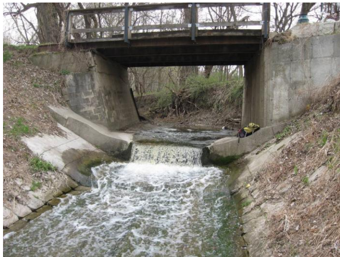
A concrete drop structure under a private driveway, pictured above, is a fish passage barrier on Picha Creek (Picture from Interfluve 2008).
