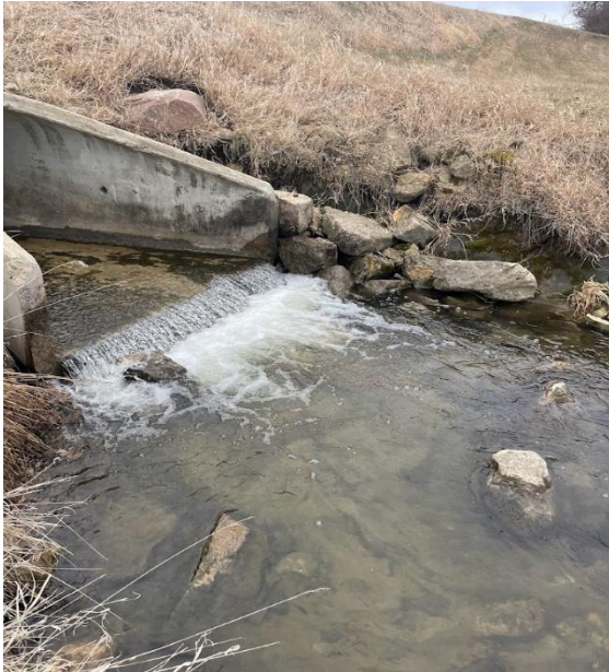
Figure 37. Perched culvert causing fish impairments at 08MN062.
