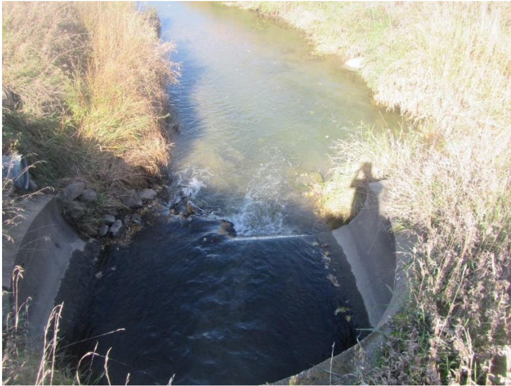
Figure 26. Perched culvert at WID -621 on Boot Creek on.
