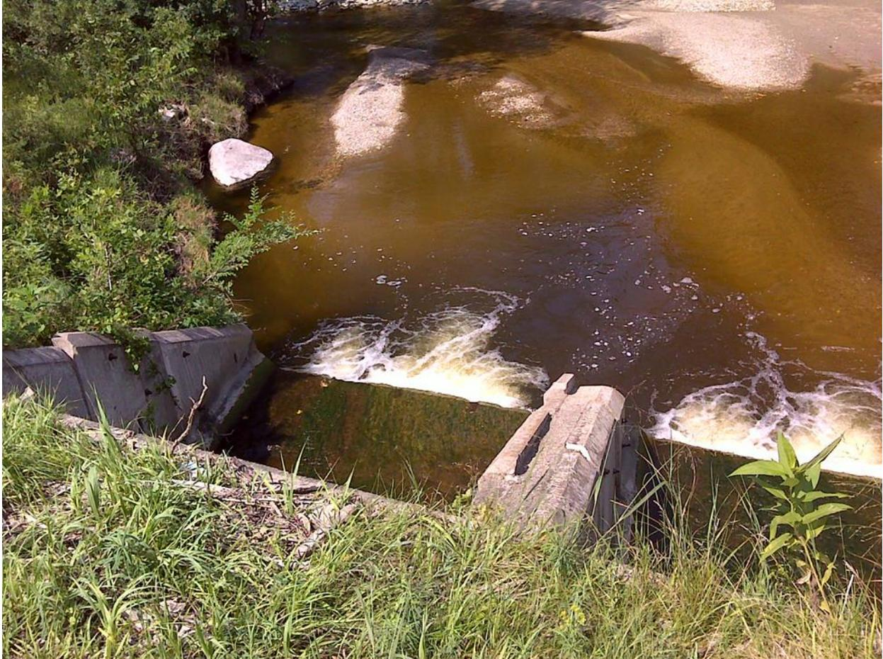
**Figure 114. Morgan Creek, Upstream of Hwy 68, on June 20, 2016, debris resting on culvert from storm event.**
