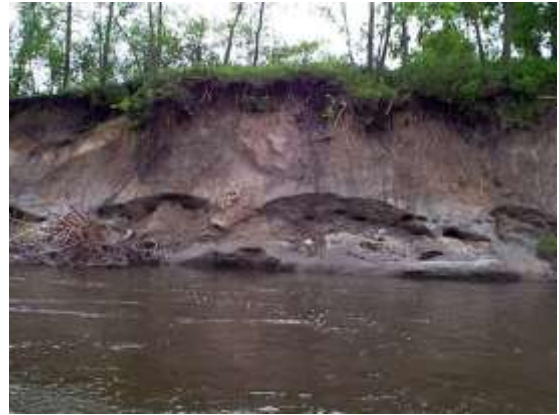
Bank sloughing a source of sediment
