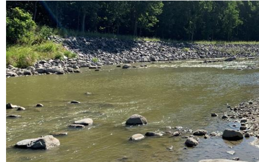
Figure 12. Bank riprap at 15MN204 (2020). Photo credit DNR.
