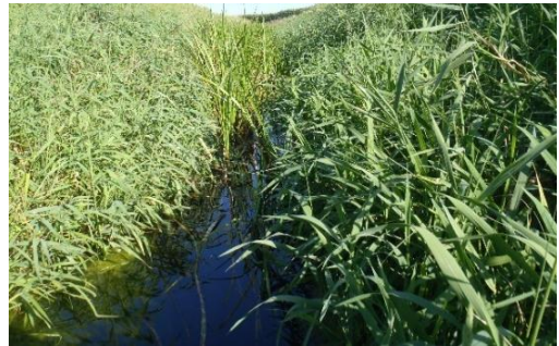
Figure 17. Vegetation filled channel at 10MN102 (7/19/10).
