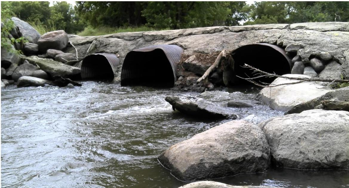
The upstream fish barrier, the field crossing is a barrier at most flows until it is inundated. The landowner is currently working on a plan to replace the crossing with a structure that does not create a fish barrier” (DNR 2019). With this culvert barrier, the upper reach of the Lac qui Parle River is not connected to fish passage from the Lac qui Parle River or the Minnesota River (Table 168). Connectivity is a stressor to reach (-515), where the culvert is located.
