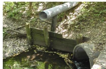
**Figure 10: Perched culvert on Long Lake Creek.**
