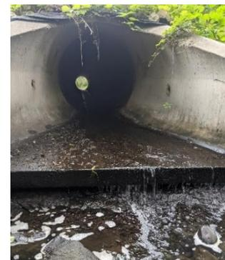
**Figure 20: Perched culvert along Fish Creek.**
