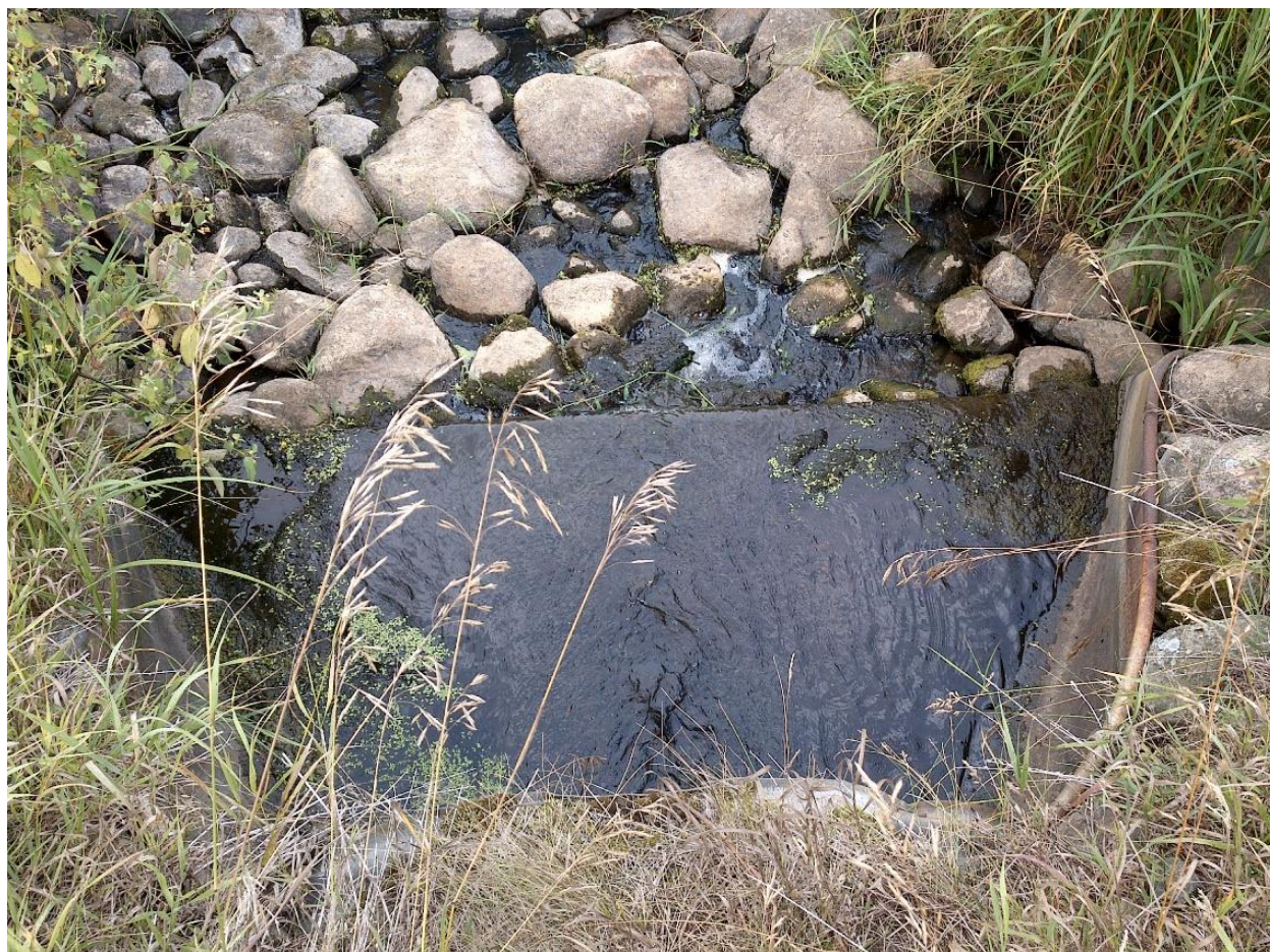
Figure 6: August 1, 2023; low flow at CR18 crossing. Drop structure at outlet and minimal water in culvert prevent fish passage.
