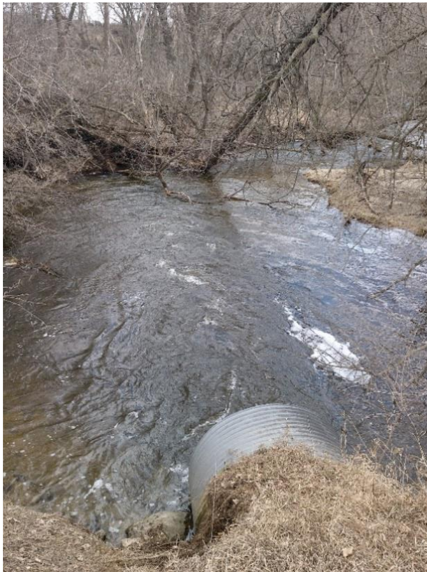
Figure 16: high spring flow velocity barrier in culvert. Water goes through corrugated metal culvert like a fire hose. Photo from 4/25/2023.
