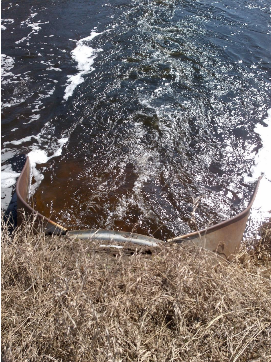
Figure 21: CD13 on 4/25/2023, showing high velocity leaving culvert.
