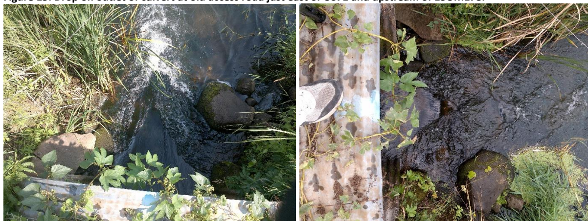
Figure 15: Drop on outlet of culvert at old access road just east of US71 and upstream of 13UM178.
