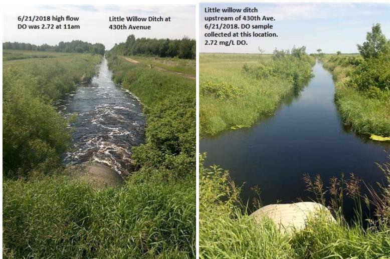
The photograph displayed here shows the high stream flow and turbulent stream velocity exiting the culvert at 430<sup>th</sup> Ave along with the upstream side of culvert where DO readings were collected.
