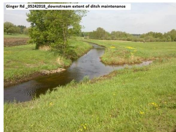
During sampling in 2016, the ditch had not been maintained very recently. Overall, it appears that not much has changed in the shape of the channel. The depth is slightly deeper and any accumulated fine sediment has been removed. By mid-summer in 2018, the channel was vegetated and appeared stable.
