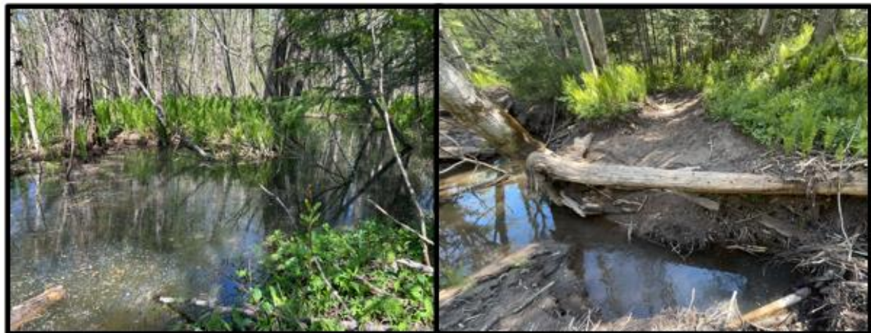
Figure 16. Beaver dam effects on Military Creek at the CSAH4 crossing include flooding upstream (left) and a disturbed channel downstream (right).
