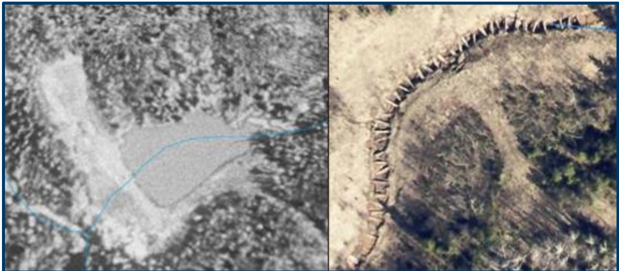
Figure 5. The failure of a 1970's dam (left) released 9000 tons of sediment to Deer Creek and a head-cut in the post-dam, restored channel (right) actively erodes sediment.
