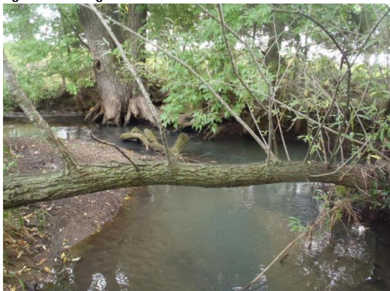
Figure 31. Eroding Streambank on the -545 reach of Threemile Creek
