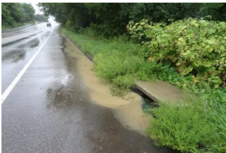
Intense rainfall carries a plume of sediment from runoff into a storm drain. MPCA photo.
