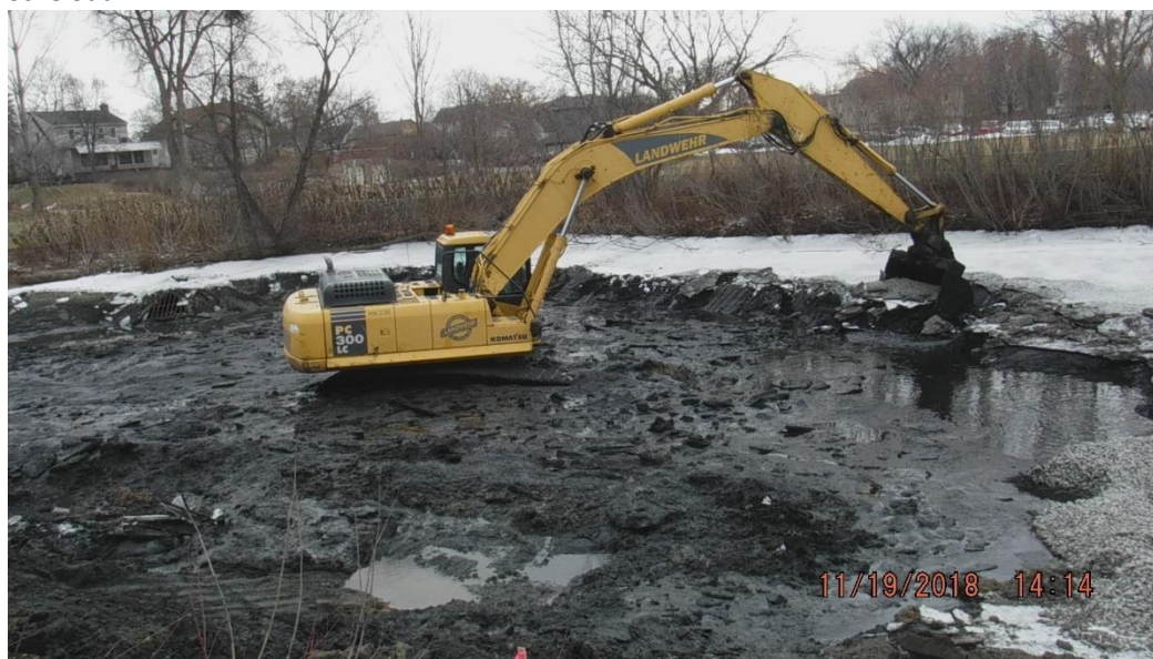
Figure 17. Dredging of the Stormwater Treatment Pond "Little George" – November 2018. Photo Credit – City of St. Cloud
