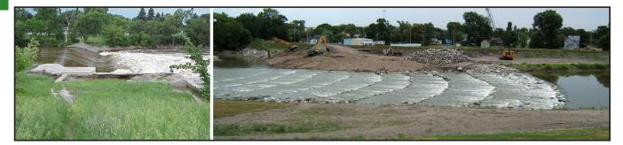
In 2005, a project involving a number of state and local watershed partners removed an old dam in Crookston (left) and replaced it with a series of rapids formed from boulders (pictured from opposite side of river). This project, along with a dam project upstream of town, restored fish passage from the Red River in East Grand Forks to Thief River Falls, a distance of 125 river miles. Fish now have access to better spawning habitat.
