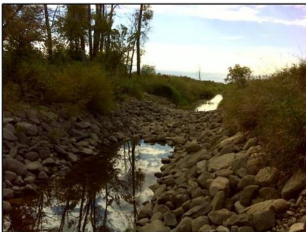
**Figure 18. Rock grade control structure possibly affecting fish passage on AUID -522.**
