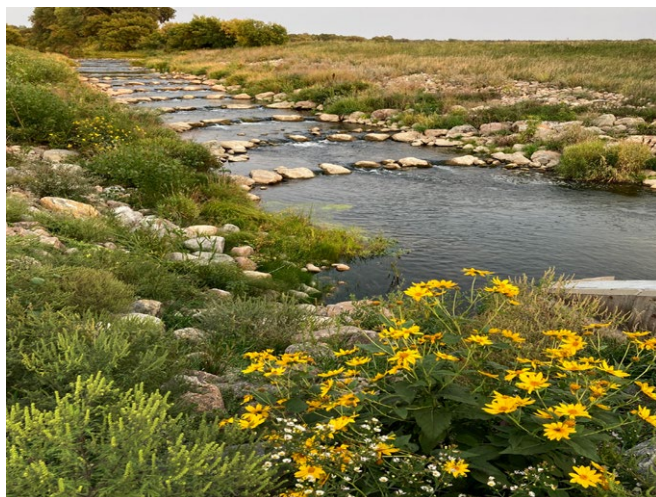
One of the riffle structures installed along the Sand Hill River. These structures replaced low head dams that previously inhibited migratory fish species from moving upstream.
