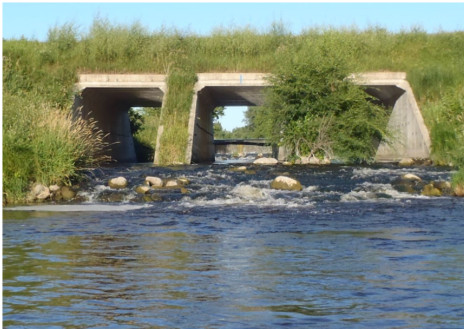
Figure 19. Image of grade control structure upstream of 11RD016 on the Sand Hill River (AUID -09020301-536)
