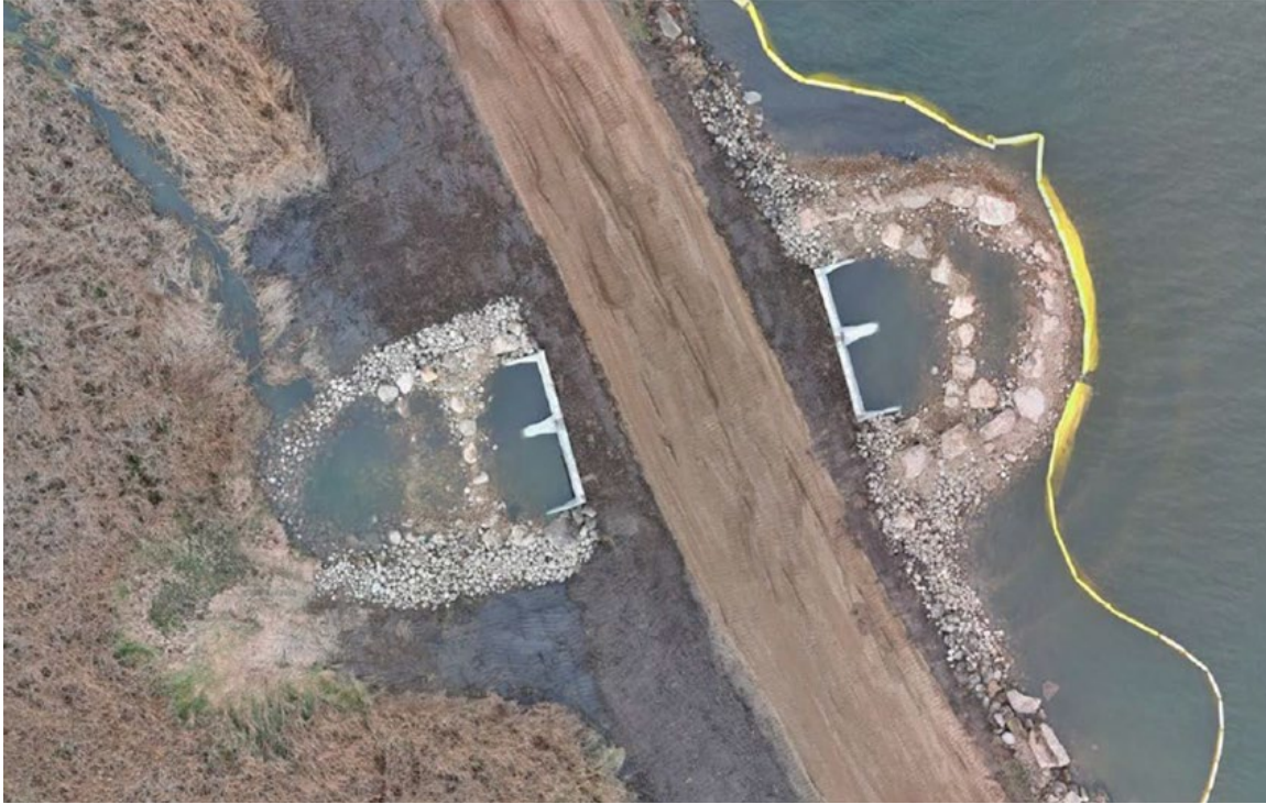
Aerial photo of the paired box culvert and riffle improvements on the outlet of Lightning Lake 11/10/2023
