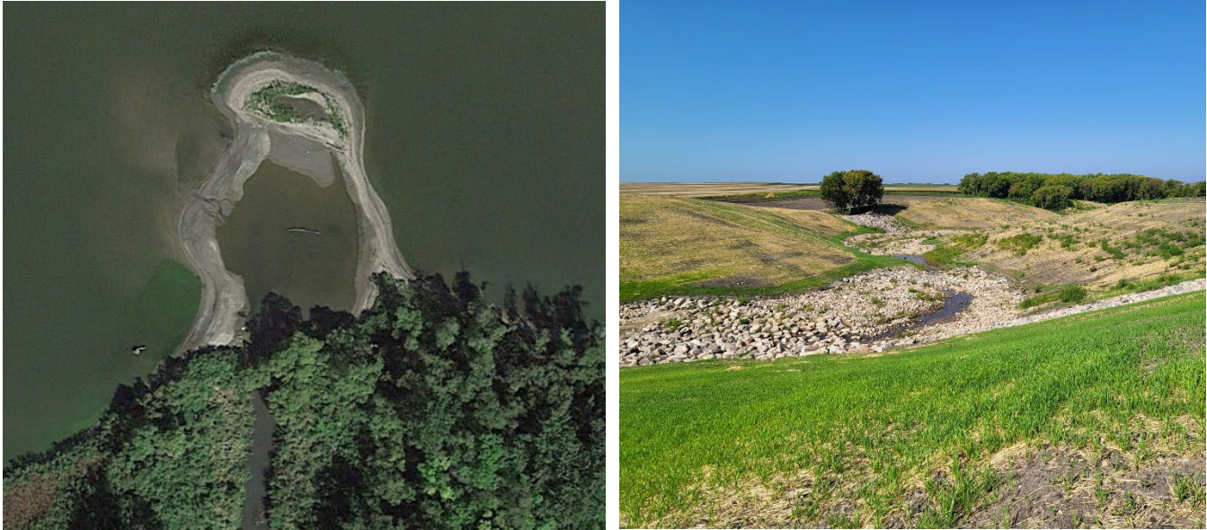
Left: Sediment plume is visible where TCD 52 meets Lake Traverse. Right: The TCD 52 above Highway 27 has been widened and armored to reduce erosion and stabilize the stream banks.
