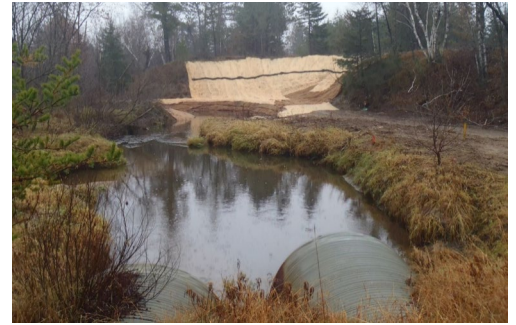
Bank stabilization efforts undertaken along Willow Creek.
