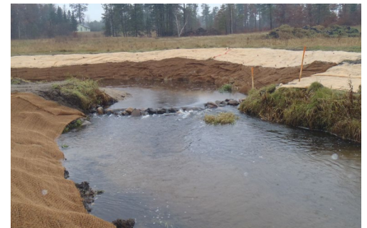
Bank stabilization and riparian restoration areas along Willow Creek.
