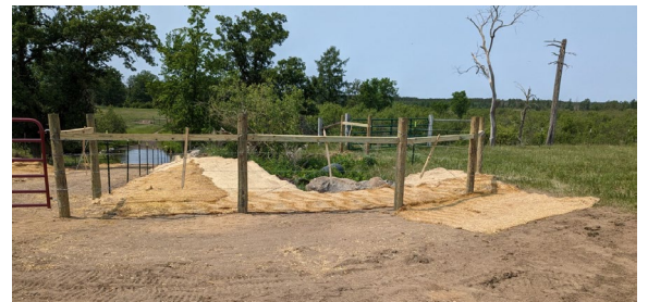
Cattle exclusion gate and fencing installed to prevent cattle from entering the river.
