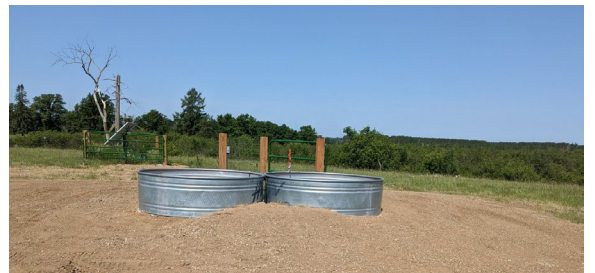
Alternative water source after completion.
