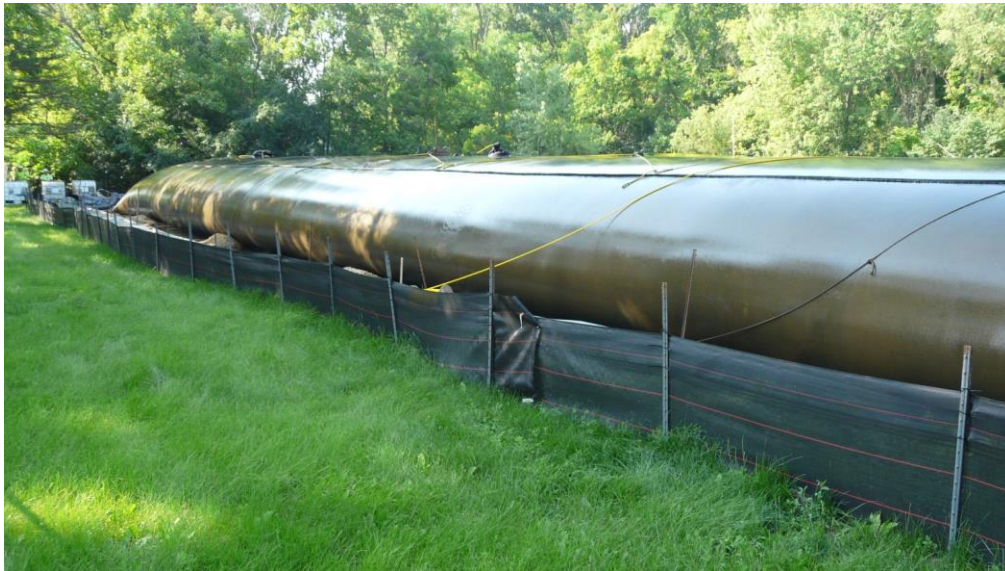
Geo-fabric bag containing stormwater sediment removed via hydraulic dredging.
