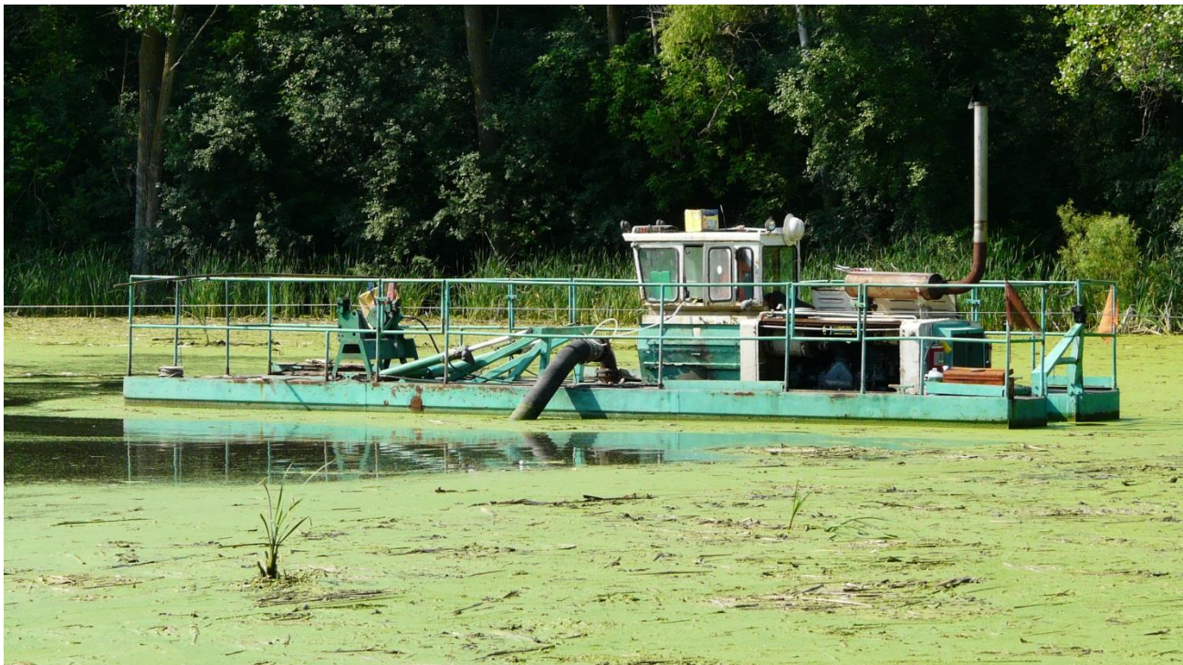
Hydraulic dredging barge in operation at Roseville Villa Park.
