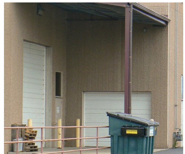
A closed dumpster and an awning over the loading dock keep significant materials from stormwater exposure.
