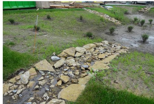
Sediment entering the basin from exposed soils on the construction site and from the side slopes **logs the system**.
