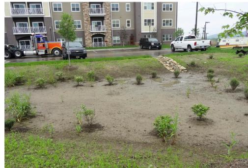
Months later, the construction project is complete. **The basin captures rainfall from a small rain event but it doesn't infiltrate**. Costly repairs are required in order for it to function properly.
