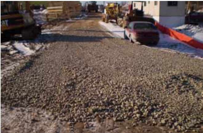
Add additional aggregate regularly to maintain a vehicle tracking pad.
