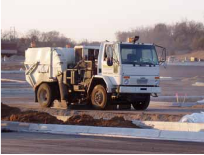
Street sweeping is required to remove any sediment that is tracked onto the street.
