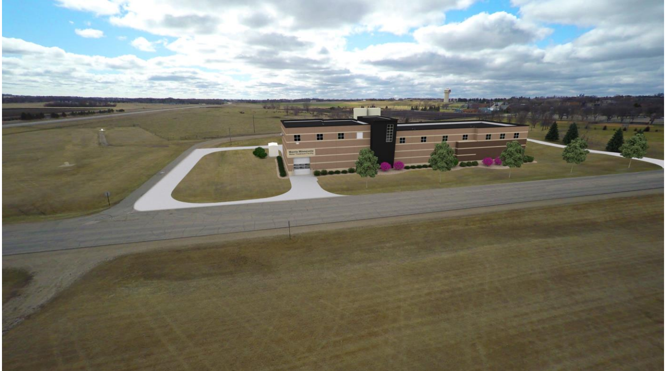
Figure 71: City of Morris Water Treatment and Central Softening Facility
