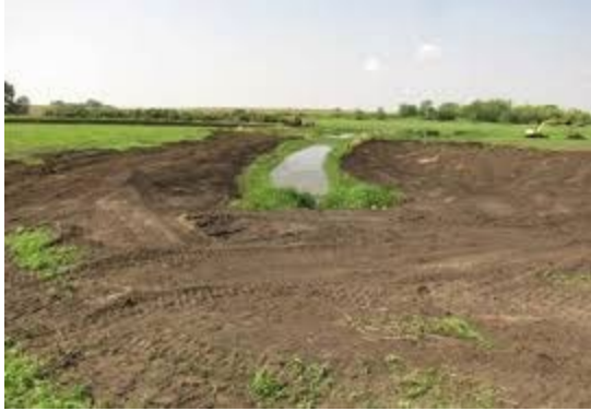
Figure 20. Example of a ditch plug. (Minnesota Wetland Restoration Guide Board of Water and Soil Resources).
