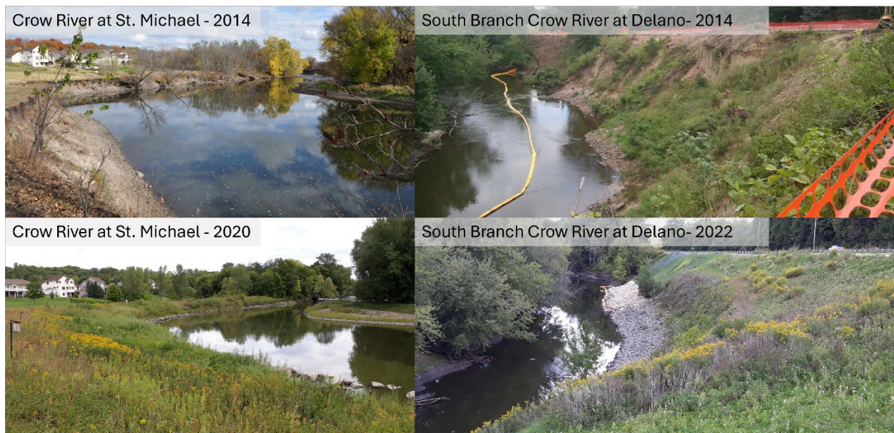
Figure 21. Bank stabilization methods; left, toe wood sod mat on the Crow River in St. Michael and, right, rip rap on the South Branch Crow River in Delano, Minnesota. During and after construction. (Photos Minnesota Department of Natural Resources).
