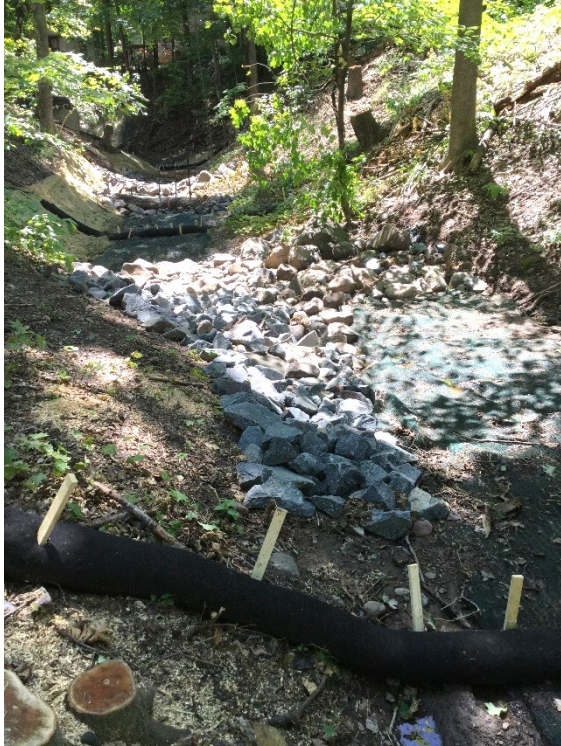
Figure 28. Check dam and rip rap stabilization method near Taylors Falls, Minnesota (photo Minnesota Department of Natural Resources).
