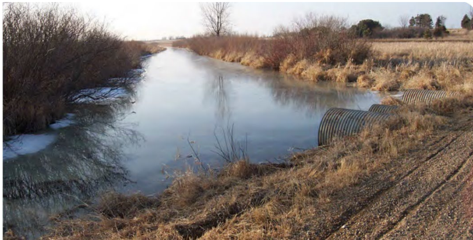
Figure 19. On-channel water storage utilizing an existing road crossing, Traverse County (Photo Ag BMP Handbook).
