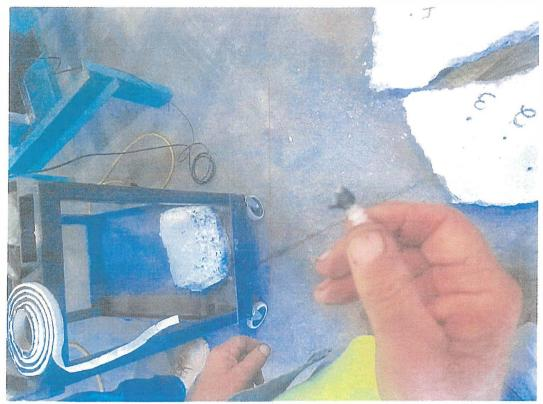
This picture shows the mastic on the plug to provide additional sealing in addition to the plug. It should be noted that the covers of all the tanks set in place via gravity with only a mastic seal and it functions well in the field.
