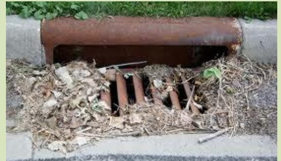
A storm drain funnels rain and snowmelt into stormwater pipes to prevent flooding. But, they also carry pollutants (like oil, deicers, and fertilizers) along with leaves and grass clippings into nearby lakes, streams, or wetlands.
