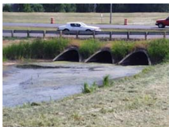
Shingle Creek Culverts, I 94
