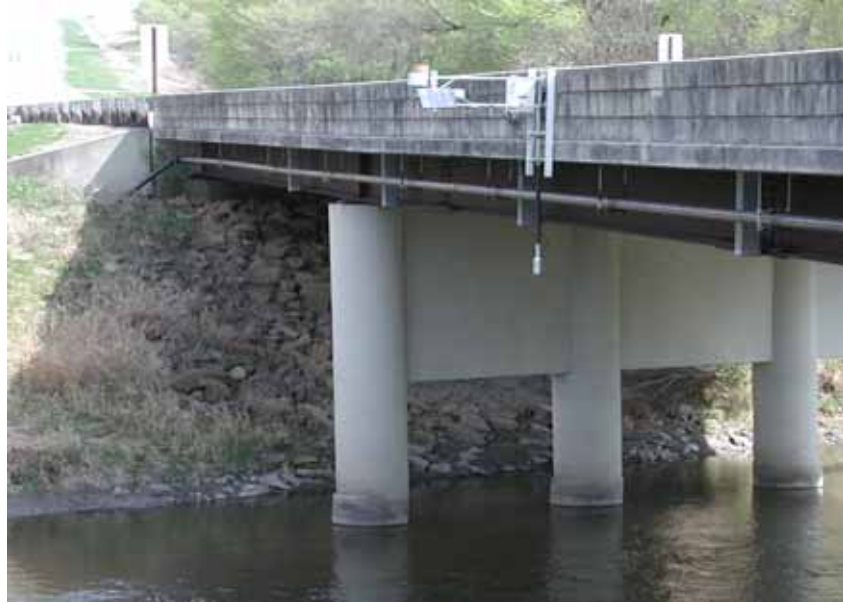
Figure 8: Bridge showing monitoring set-up
