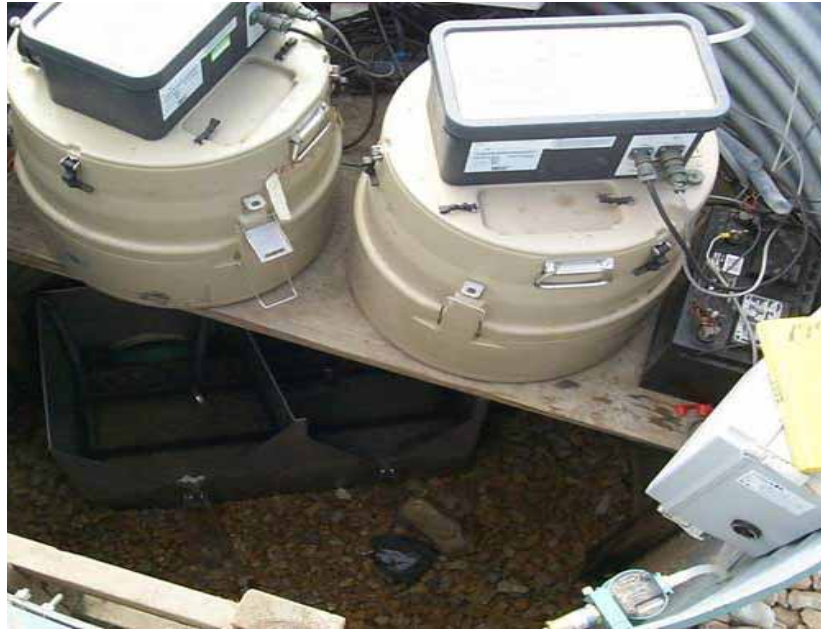
Figure 10: Stilling Well with Automated Sampling Equipment
