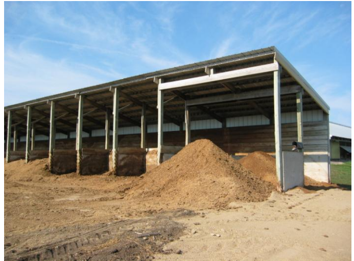
Turkey compost shed
