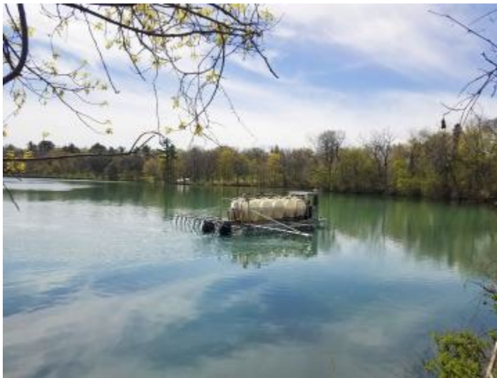
An alum treatment in progress on Sunfish Lake, used to make less phosphorus available to fuel algae growth.
