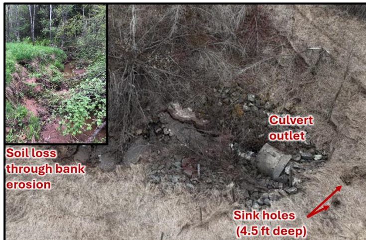
Figure 9. Soo Line Trail culvert outlet at Elim Creek. Two sink holes have formed near the outlet and there is evidence of eroding and undercutting banks and channel incision.
