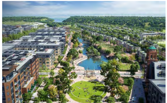
Figure 16. As part of the Ford Motor Assembly Plant redevelopment, the City of Saint Paul used Clean Water Funds to create a stormwater treatment system as part of a central water feature that filters stormwater runoff from more than 60 acres and removes 75% of phosphorus and 94% of total suspended solids (TSS) prior to discharging into the Mississippi River. This innovative biofiltration project will clean 64 million gallons annually, preventing an estimated 145 pounds of phosphorus and over 55,000 pounds of total suspended solids from reaching the river while creating an amenity surrounded by green space that will provide multiple types of recreational opportunities for the community.
