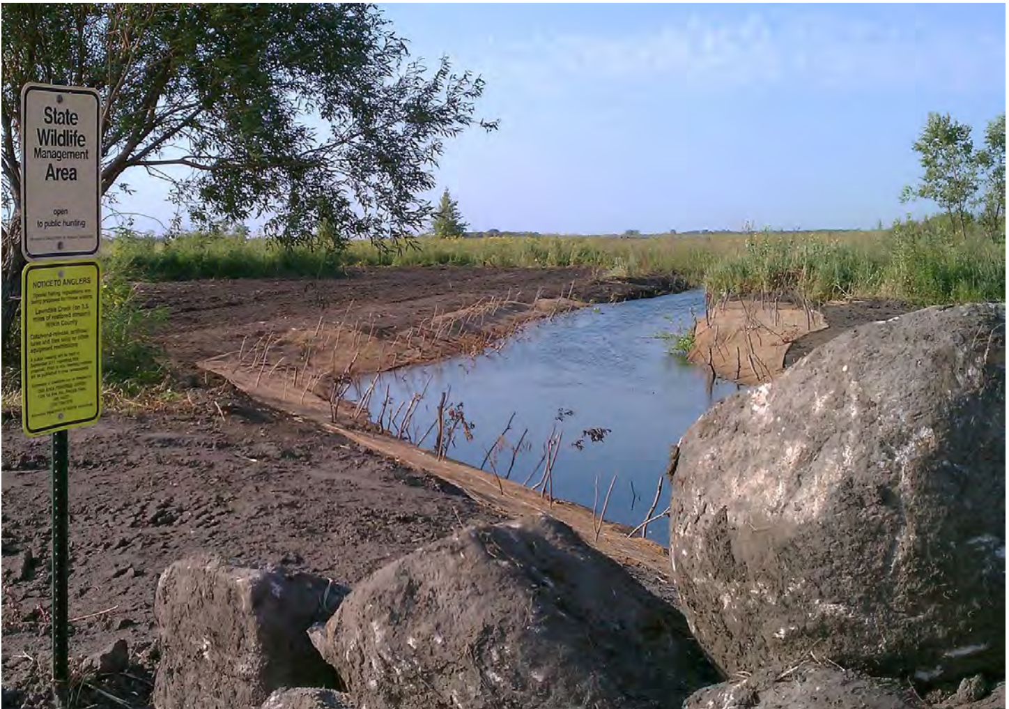
Figure 29. Local organizations restored Lawndale Creek's naturally meandering channel to reduce erosion and improve habitat in the trout stream in the Buffalo River Watershed.
