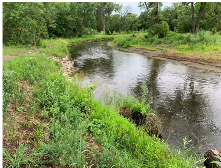
An expansive project to integrate water quality and habitat improvements into an overhaul of Edina’s Arden Park includes a remeandered portion of Minnehaha Creek (above) and a new regional stormwater management system that involves an underground pre-treatment structure and six biofiltration swales planted with native plants (below).
