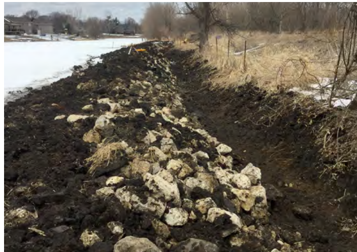
Vegetated riprap helps to stabilize the streambanks and control erosion. Photo Courtesy of Lakeville city staff
