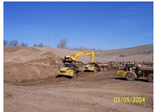
*Subgrade excavation for cell construction at the Elk River Landfill.*
